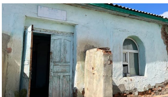
Figure 15 Sign and entrance door of the Mosque complex. Photo by naMec, 2024.
