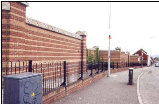
Fig. 3. Torrens Avenue (June 2 nd , 2001) © F. Ballif.
